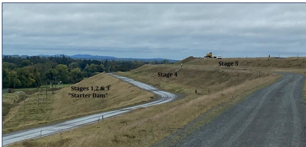
Figure 5.2 Existing Embankment side profile
